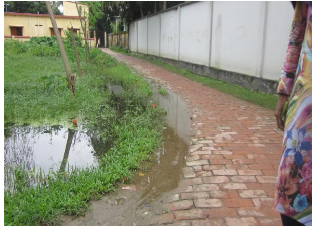
View of road PDP-202
