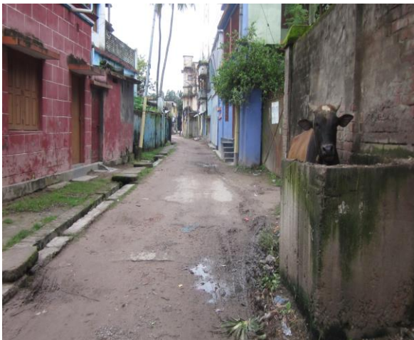
View of drain PDP-79
