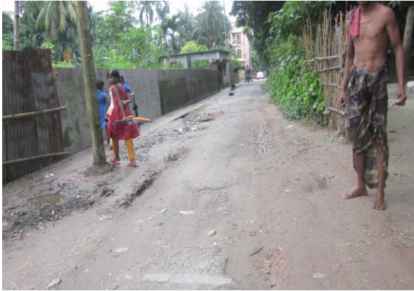
View of road PDP-98
