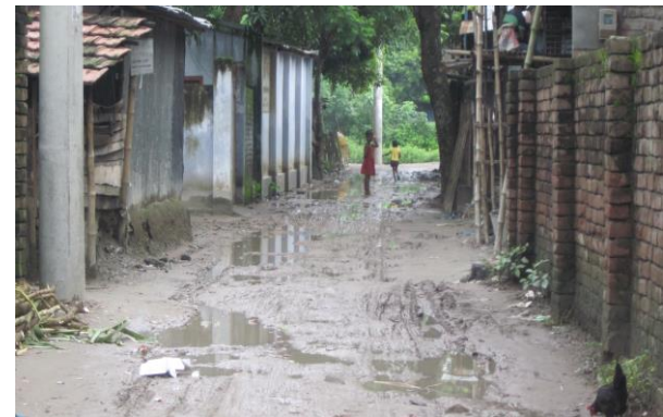
View of road PDP-191
