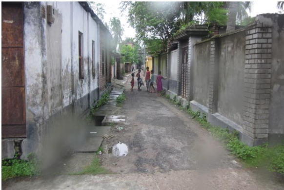
View of drain PDP-28
