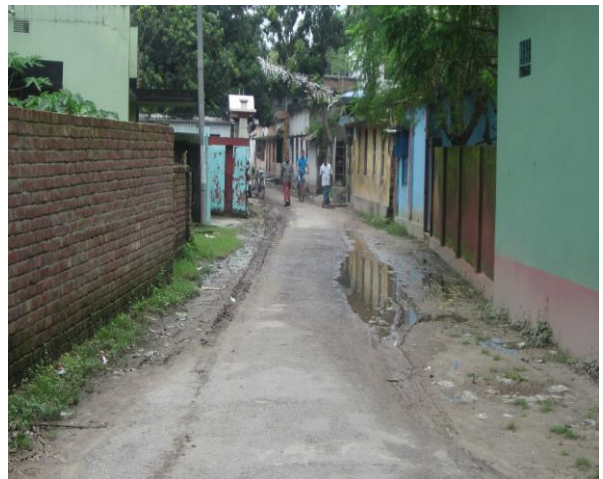
View of drain PDP-26
