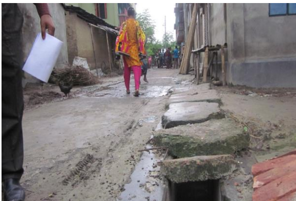
View of road PDP-159
