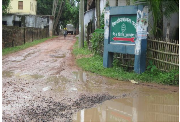
View of road PDP-98
