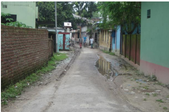
View of drain PDP-147
