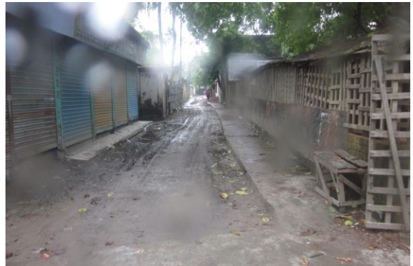
View of road PDP-164
